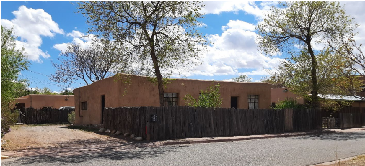
Residential building across Alto Street (Southeast)
