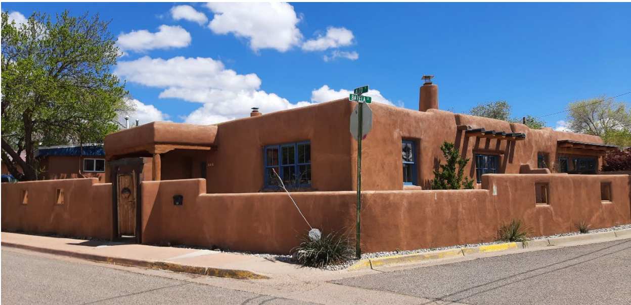
Residential building across Alto Street (Southwest)
