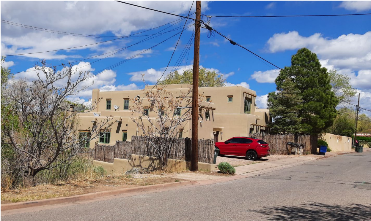
Adjacent residential compound from Alto Street (West)
