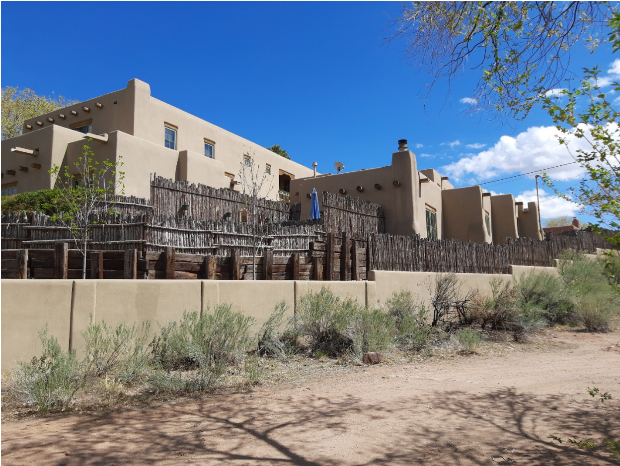
Adjacent residential compound (West):
